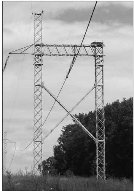
Figure 1: Bald eagle nest on transmission tower in western Minnesota.
