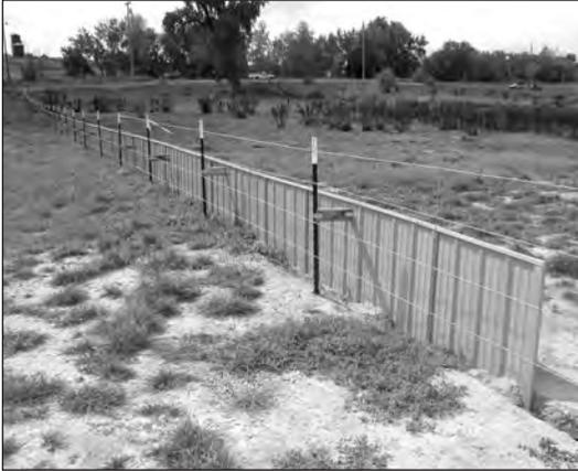
Figure 2. A corrugated steel barrier, partially installed.
