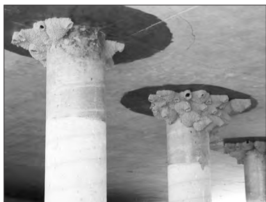
Figure 7. Completed nests on piles and overhead surfaces treated with silicone paint.
