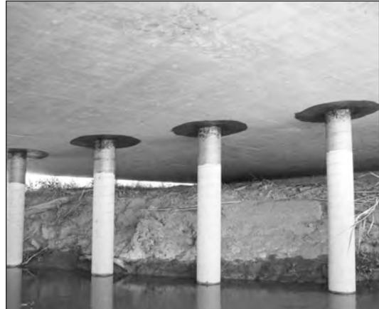
**Figure 4.** Highway structure with silicone paint surface modification.
