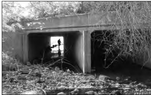
Figure 1. Large double culvert.
